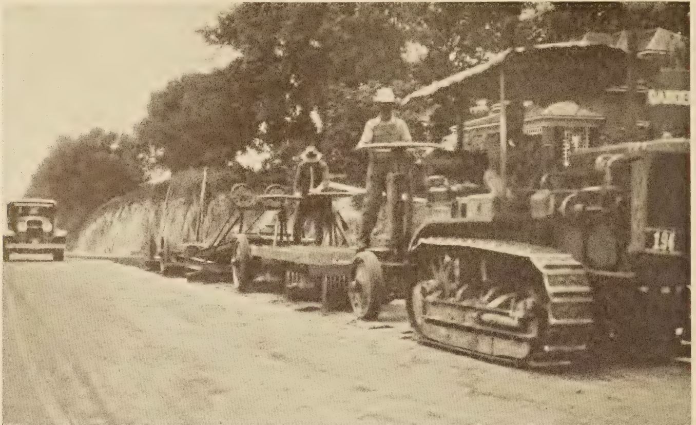
FIGURE 9.—PREPARATION FOR RETREATMENT: TRACTOR HAULING SPECIAL DISK PLANER AND MULTIPLE-BLADE MAINTAINER
